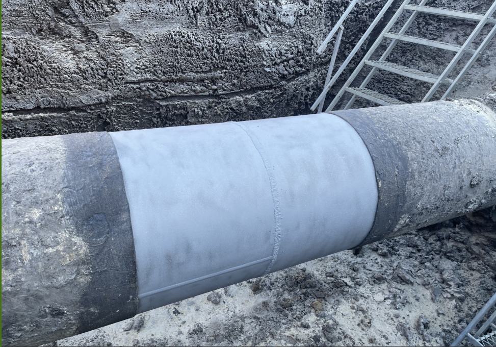
Defect weld grit blast and cleaned with acetone
