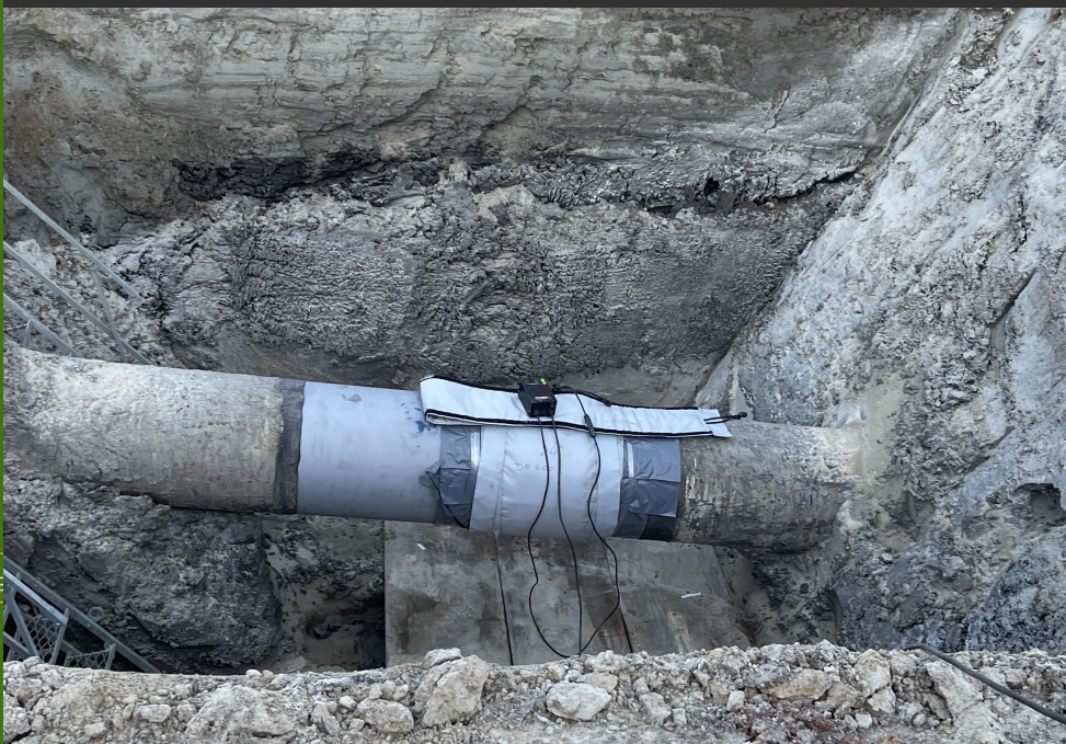
Repair installed below freezing so cured under a heat blanket
